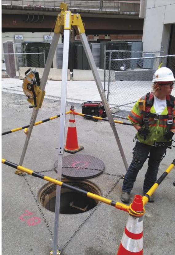
Dangerous confined space entries are made safe with the right personal protective equipment and safety measures.
